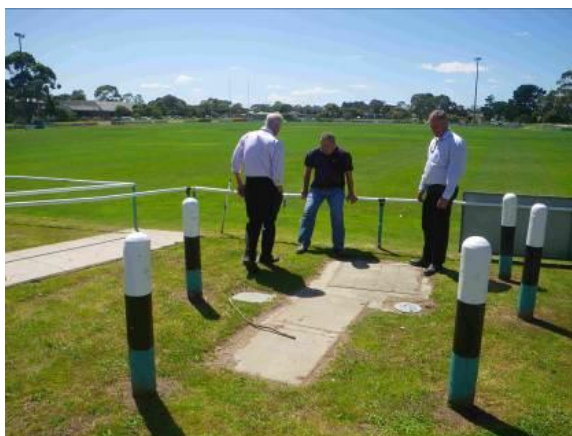
Figure 6 – Existing irrigation header tank
