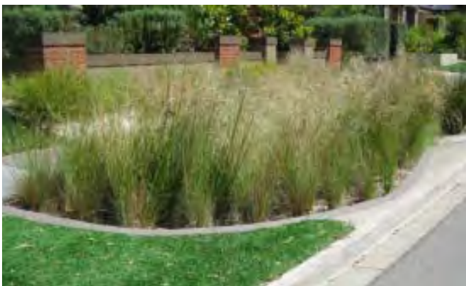
Healthy, densely planted vegetation is important to the long-term performance of the raingarden.
