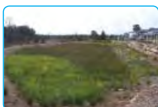
d) Bio-retention basin / raingarden
