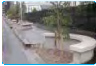
a) Street tree bio-retention system
