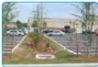
b) Bio-retention swale
