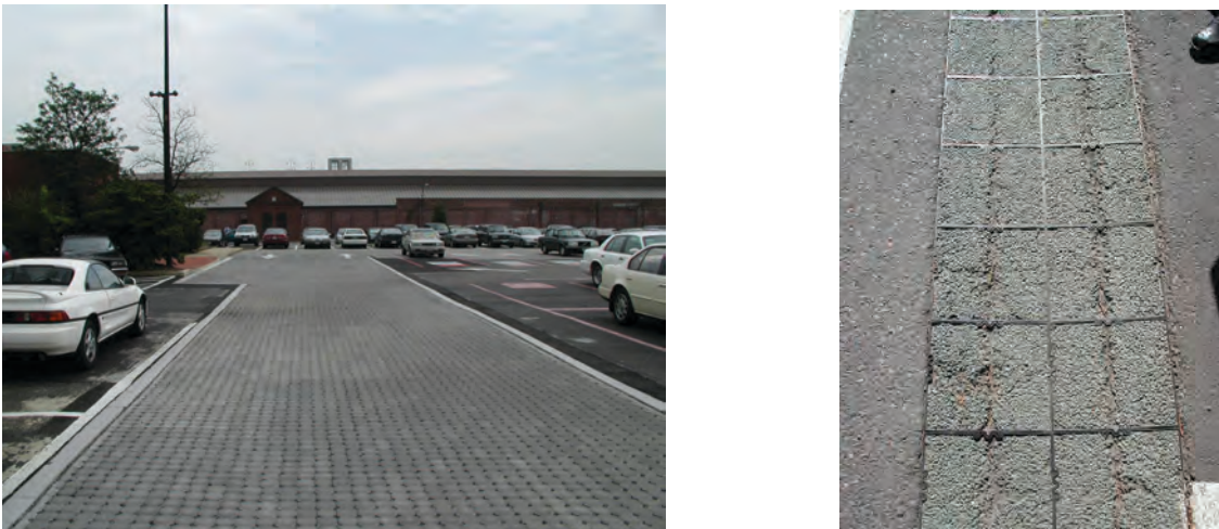
Figure 14.2 Examples of porous pavement: porous car park, Washington, DC, USA (Photo: Ecological Engineering); porous car park, road gutter, Manly, NSW (Photo: Tim Fletcher).
