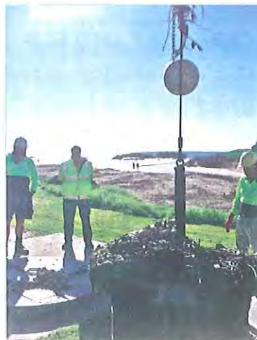
Basket cleaning of a CDS GPT.
