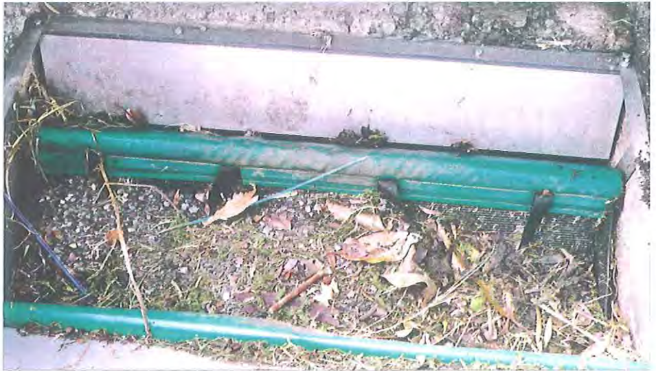
A pit basket that is full and overdue for maintenance.
