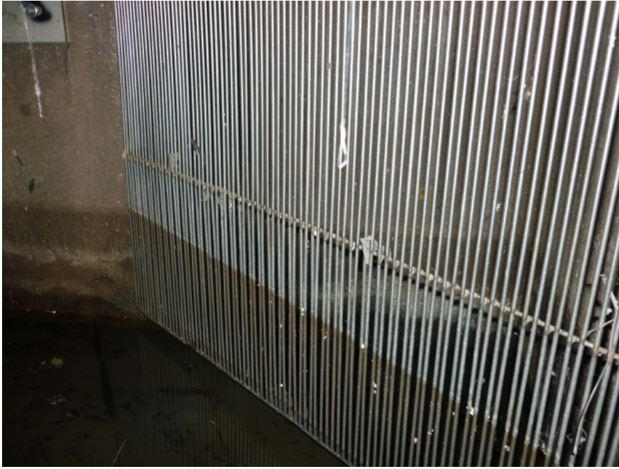
A Humegard screen cleaned and ready for action.
