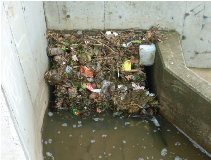
The design of the offtake into this undersized GPT is very poor. This photo was taken one week after cleaning. Exclusion bar design can limit GPT functionality if not done well, and be a maintenance nightmare
