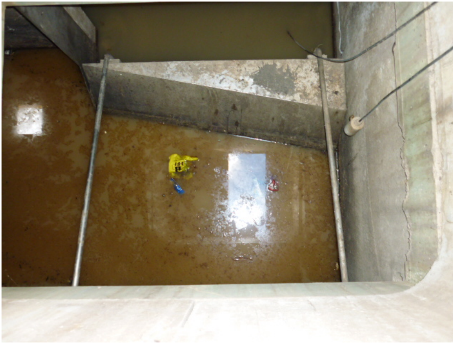
Backwater in this Humegard complicates the cleaning process, because it must be suction cleaned
