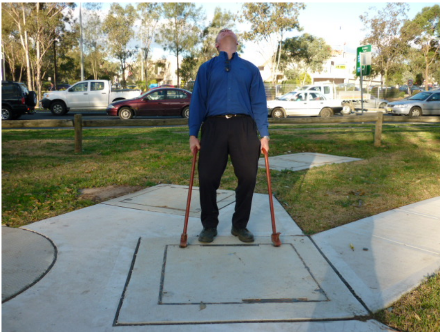
Some lids can be so heavy that they do not comply with workcover requirements to open them, or like this one, cannot be opened at all.
