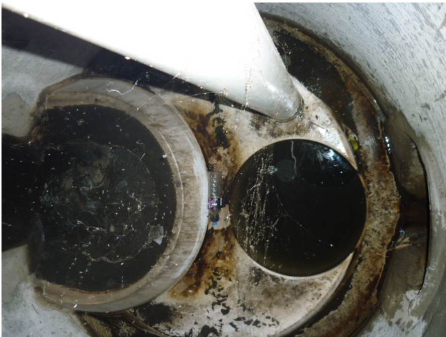
The inlet on this Humeceptor is blocked and requires cleaning to reinstate the device to operational
