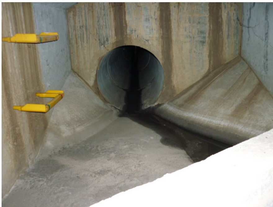
A correctly installed and well maintained diversion chamber
