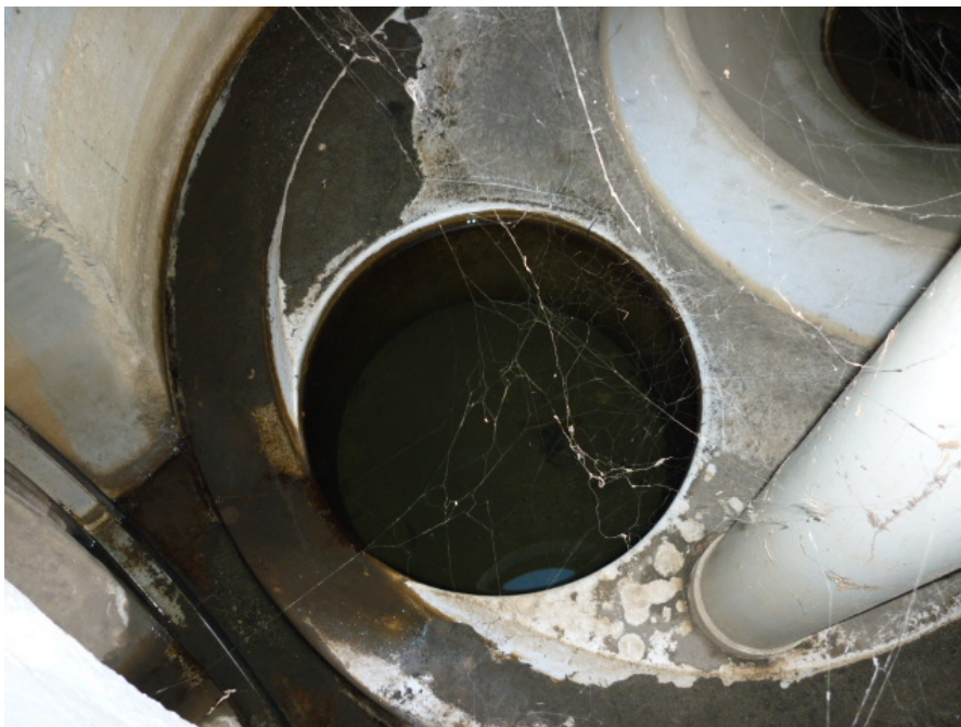
This Humeceptor has considerable sediment deposition on the fibreglass insert, and requires a thorough clean
