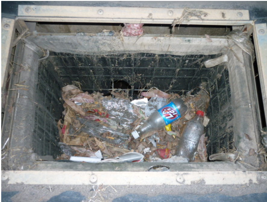
The mesh in this Enviropod Pit Trap is too fine. The mesh is also torn and there is pollution stuck on the overflow supports suggesting pollution is bypassing. Use of coarser mesh is suggested, plus more regular inspection and cleaning
