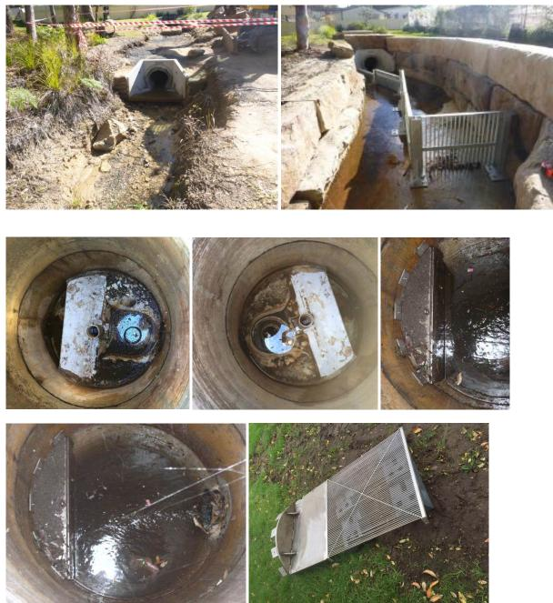
Optimal Stormwater provided the rectification design which involved enhancing the Humeceptor into a baffled screening system, which would then protect the pump and be much much easier to clean.
