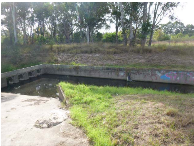
Figure 12 custom trashrack sediment sump and offline storage bay
