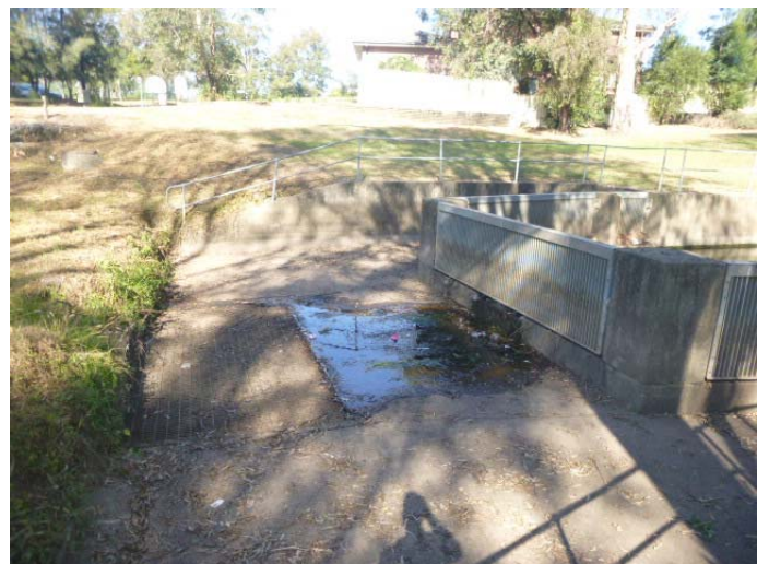
Figure 12 custom trashrack sediment sump and offline storage bay
