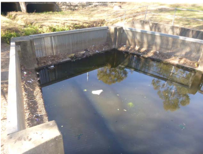
Figure 12 custom trashrack sediment sump and offline storage bay
