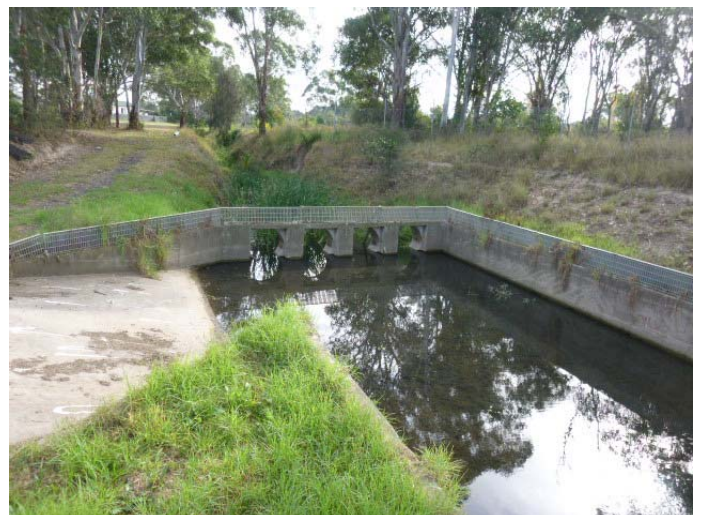
Figure 12 custom trashrack sediment sump and offline storage bay
