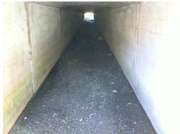
Figure 2 - Downstream culvert, under a major RTA road.
