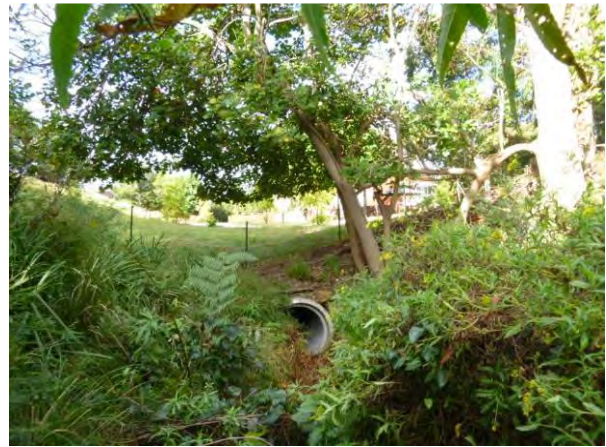
Figure 5 - Downstream the inlet structure
