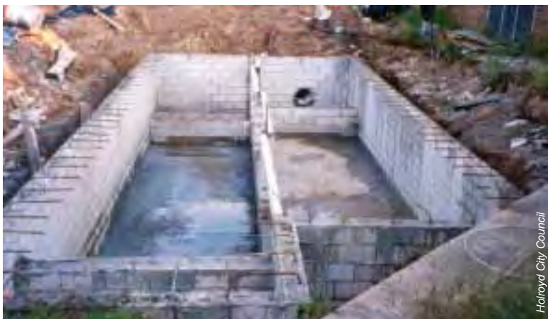
Sand filter under construction (showing sedimentation and filtration chambers)
