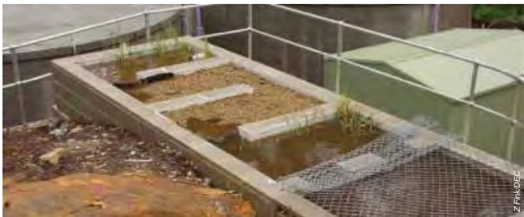
Sand filter and wetland
