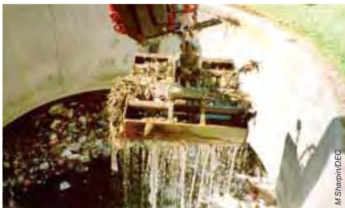
Trash removal, Centennial Park
