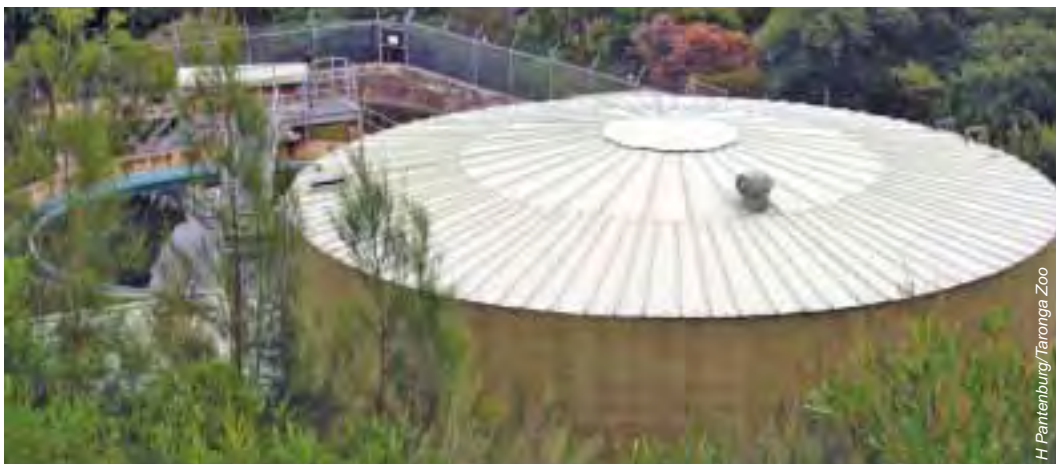
Taronga Zoo stormwater and wastewater treatment plant
