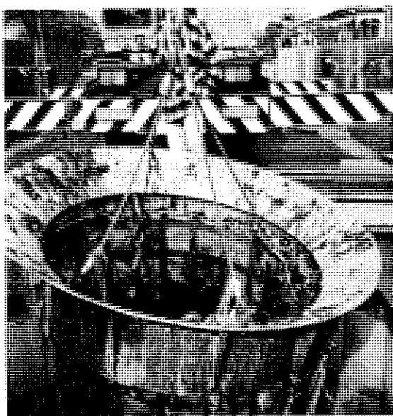
Figure 8.10 Buckets located in cranes are also used to collect pollutants, and are removed by crane. Coburg, Victoria (source: R. Allison)
