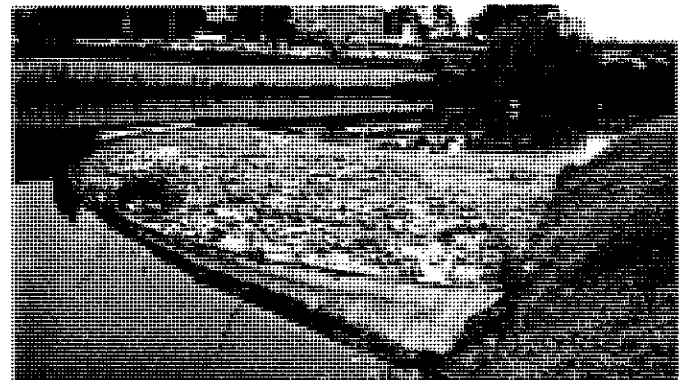
Figure 8.21 Early designs of floating traps were based on oil retention booms and prone to wind scour of collected pollutants. Richmond, Victoria (source: R. Allison)
