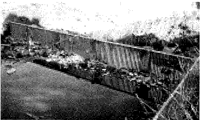
Figure 8.17 Direct screening devices can be prone to blockage and overtopping. Broadmeadows, Victoria (source: R. Allison).
