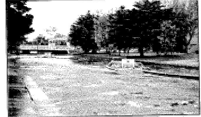
Figure 8.23 Floating traps can be subjected to high forces and velocities during flood events that can compromise their structural integrity. Elwood, Victoria (source: R. Allison)
