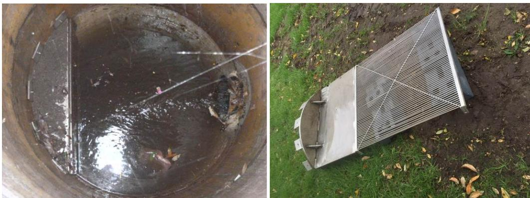
Optimal Stormwater provided the rectification design which involved enhancing the Humeceptor into a baffled screening system, which would then protect the pump and be much much easier to clean.
